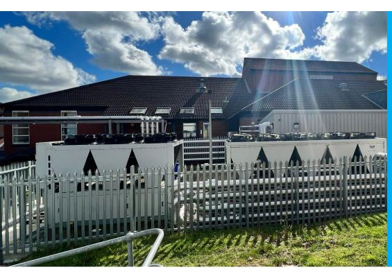
ICS Cool Energy multi-pipe chillers and heat pumps took over from the hospital's gas boilers, reducing heating system's gas consumption by almost
