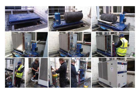
• Dismantle and Reconstruct – Flat pack assembly where there is minimal access, we can deliver our equipment in kit form, and then rebuild on site.
